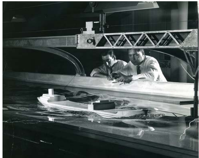
Daniel Savitsky (R) and Pierre deSaix during 1965 tests of a 550 ft (168 m) tanker in the Davidson Laboratory (Photo courtesy Davidson Laboratory, Stevens Institute of Technology)
