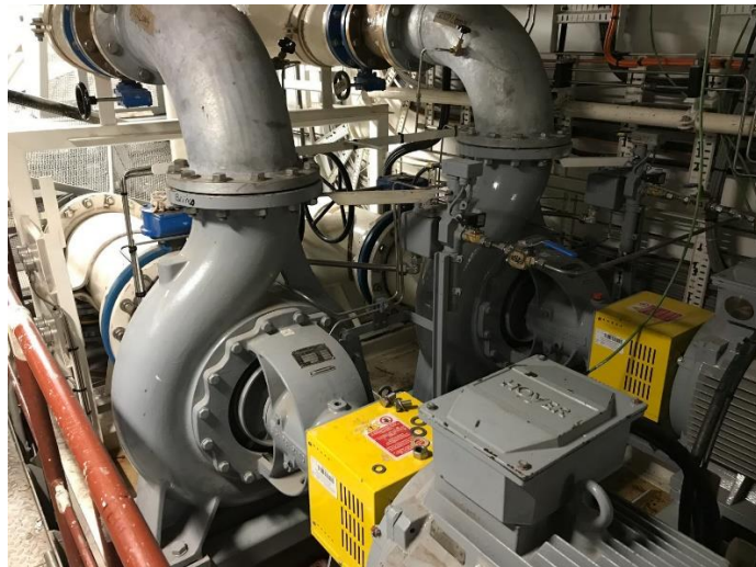
Nuyina's drain pumps for the wet well sampling space (Photo courtesy Australian Antarctic Project)
