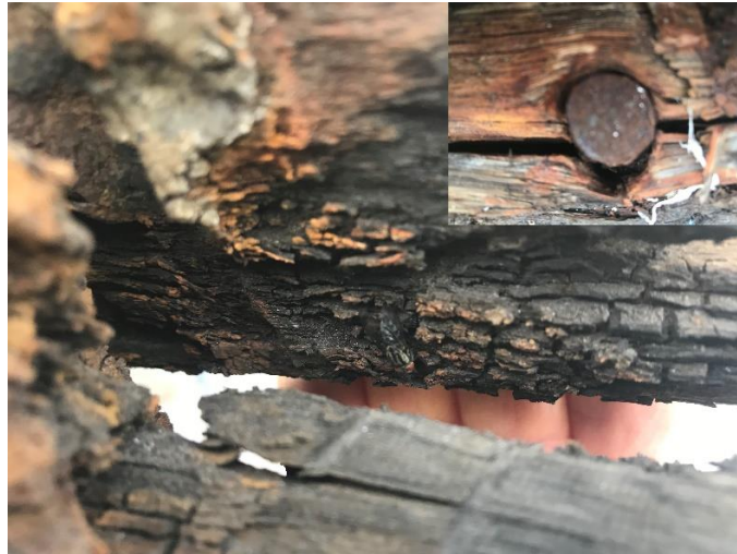
Electrolytic rot (Photo courtesy Noakes Group)
