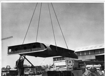
The 45 tons travelling crane has an auxiliary hoist which in conjunction with the main hoist enables large sections to be turned over without the aid of another crane and as the turning process is performed in mid-air the necessity of providing turning pits to accommodate projections is obviated.
