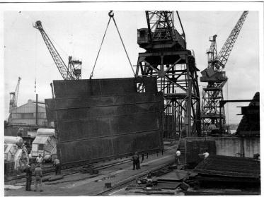
Complete Bow and Stern Units, side shell panels and double bottom units etc. which are beyond the capacity of the shop cranes are prefabricated on the assembly areas within reach of the 45 tons travelling crane. The final assembly and welding together of smaller components prior to erection on the Building Berths is also carried out.
