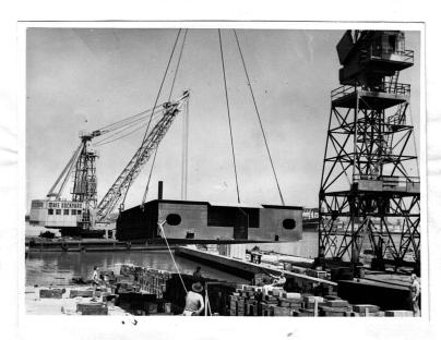
The Keel or more correctly the midship double bottom unit was erected on the building berth on 11th November, 1954.
