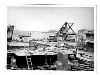
No jigs are used in fairing the shell panels, but a rather novel method of fairing by means of the erection and "winding in" of steel waterline offset battens has proved very successful.
