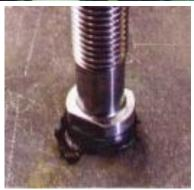
Welding 20mm studs in the moon pool of Chevron's Genesis platform for replacing riser bumpers.
