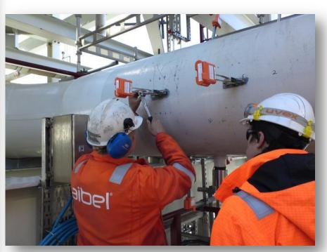
Friction welding procedures were qualified using the explosive atmosphere test with the explosive gas mixture inside the pipe as well as surrounding the weld for pipes carrying hydrocarbons.
