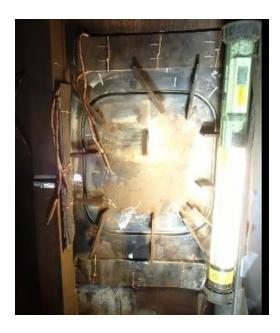
The access window closed and re-welded
