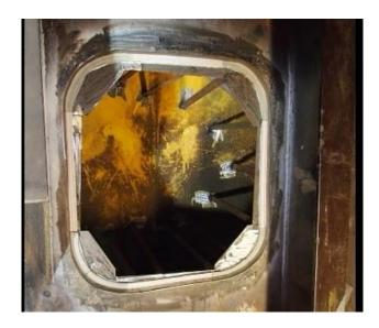
Access window cut in the FPS hull after the cofferdam was attached
