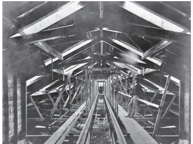
Froude towing tank at Torquay.
