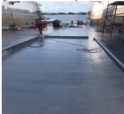
The pontoon deck replated (Photo courtesy Noakes Group)
