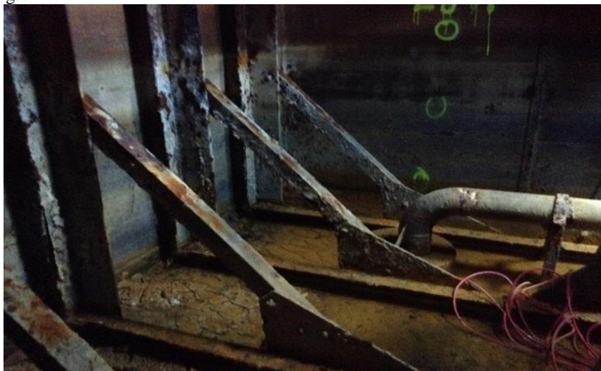
Poor condition of internal tank paint (Photo courtesy Noakes Group)
