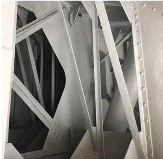
Repaired and repainted internal structure (Photo courtesy Noakes Group)
