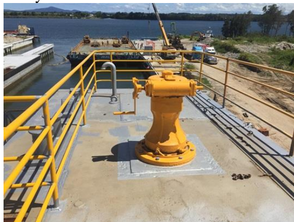
New handrails and rebuilt capstan (Photo courtesy Noakes Group)
