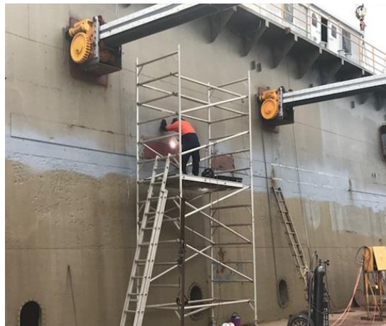
New side shores and refurbished drive motors (Photo courtesy Noakes Group)
