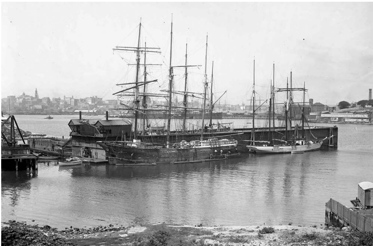
The Victoria Jubilee Floating Dock, named in honour of Queen Victoria, was located in Cameron's Cove, in the Sydney suburb of Balmain. The dock was designed and built by James Anderson of Anderson, Goodall & Co. of Balmain. It was 97 m long, 17.3 m wide and 8.2 m deep with displacement of 14 763 t. The dock received its first ship, Royal Tar , on 1 October 1887 (Photo Australian National Maritime Museum Collection)
