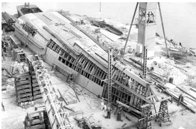
The lower forebody units for HMAS Voyager under construction in May 1949 (J C Jeremy Collection)
