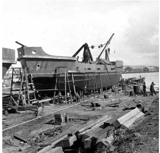
A 36.4 m cargo vessel under construction for the US Army Transportation Service; these ships were all welded (John Jeremy Collection)
