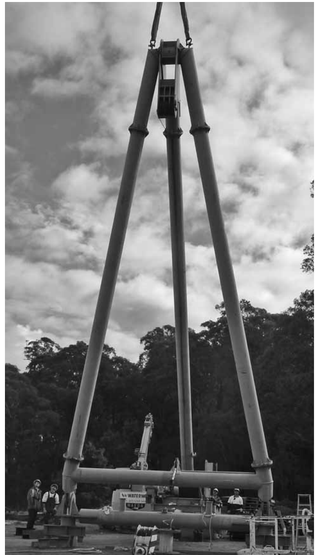
Sheer legs on 27 m barge (Photo courtesy BCTQ)
