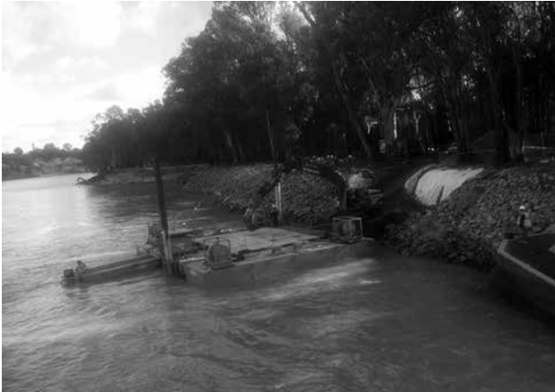
Transfer of earthmoving equipment onto a pontoon (Photo courtesy BCTQA)
