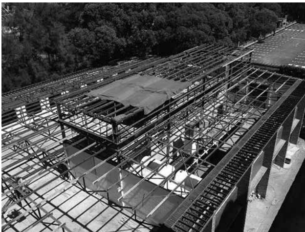
Roof of Willis Annex South, showing the encapsulation of the existing wind tunnels in the Aerodynamics Lab for protection during works (Photo courtesy Tracie Barber)
