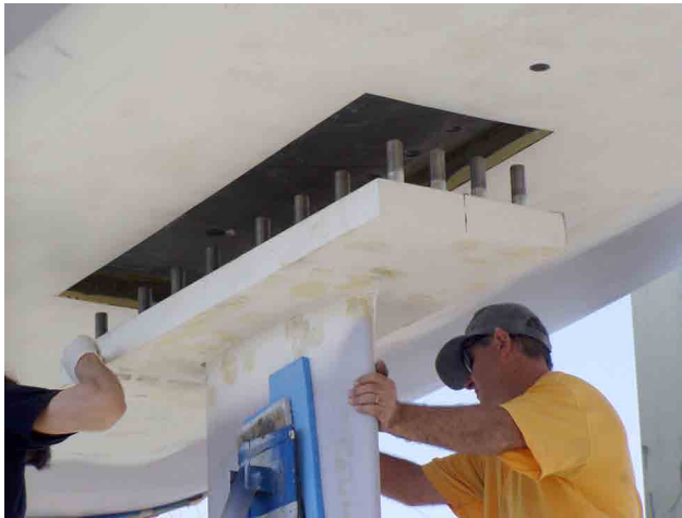
Keel flange and bolt arrangement on the Vanguard 60 (Photo courtesy David Lyons)
