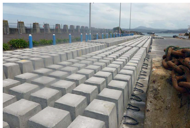
Mattresses ready for deployment on the harbour bed at Eden (Photo courtesy Robert Whiter)
