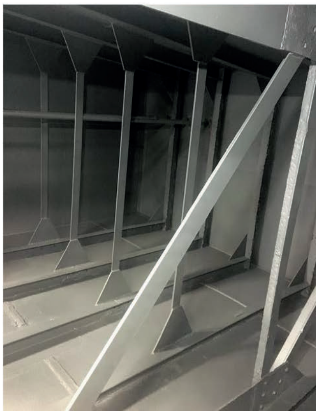
Repaired and repainted internal structure (Photo courtesy Noakes Group)
