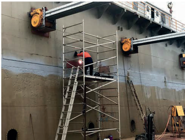
New side shores and refurbished drive motors (Photo courtesy Noakes Group)
