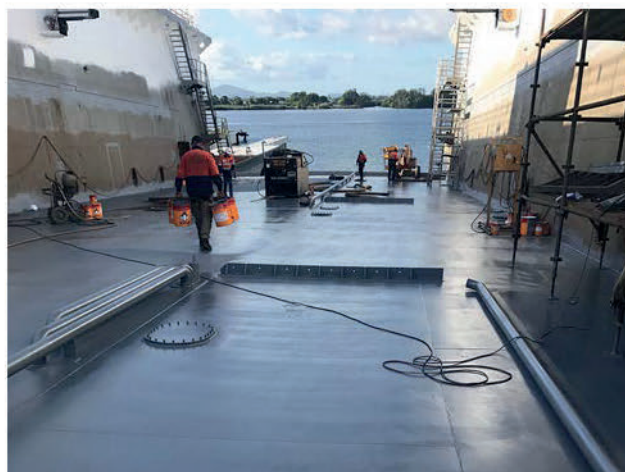
The pontoon deck replated (Photo courtesy Noakes Group)
