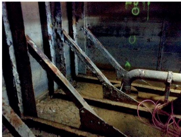
Poor condition of internal tank paint (Photo courtesy Noakes Group)
