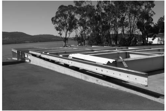
Austal's Crandall slipway for launching vessels at Margate (Photo courtesy Anne Simpson)
