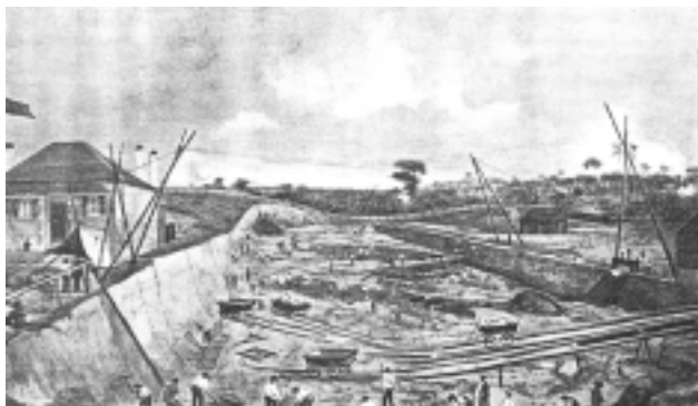
Excavation work for the graving dock (from Mort's Dock, Fifty Years Ago and Today )
