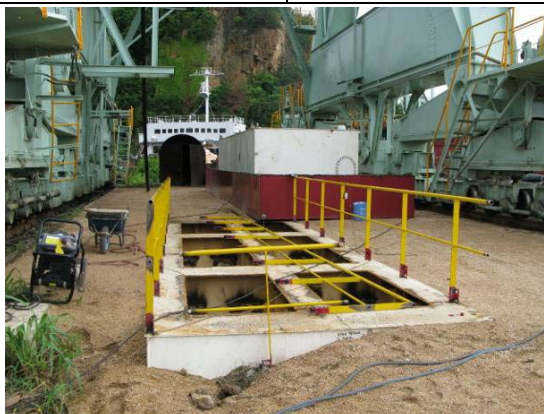
Drain system to control contaminated soil by providing rain pit
