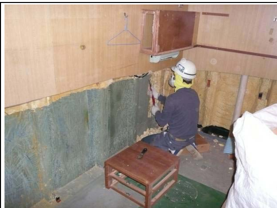
Removing flammables along the cutting lines before gas cutting (pre-cleaning work)
