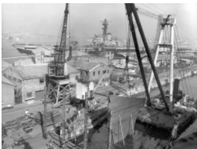
Placing the new bow unit in dock during the 1969 repair (Cockatoo Dockyard photograph, J. C. Jeremy collection)
