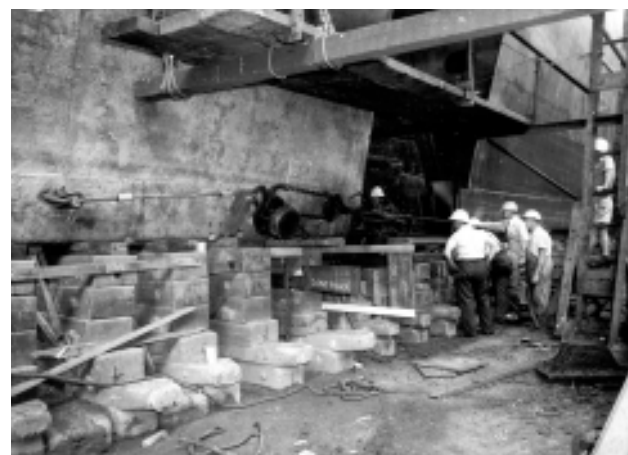
The bow unit being hauled into position (Cockatoo Dockyard photograph, J. C. Jeremy collection)
