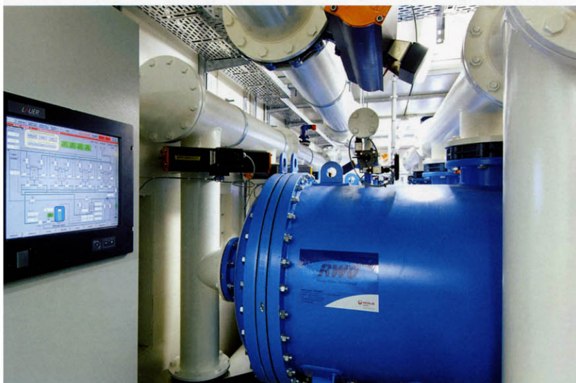
The CleanBallast system for ballast water treatment in the land-based field test.
